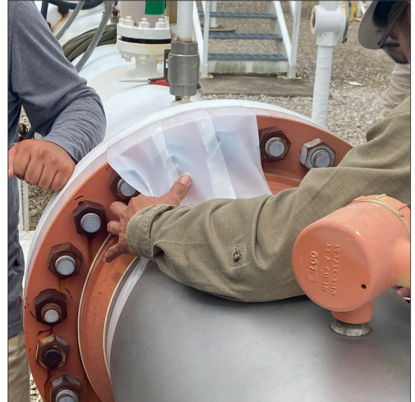
Application of ZERUST® ZIF Tape for Internal Flange Protection on a 24-inch Pipe Section.
